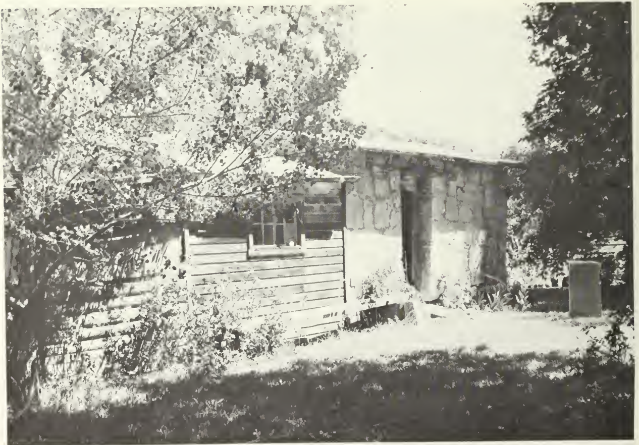
Photo 36. South side of stone house showing frame addition in 1978. (Photo Credit: Bureau of Land Management).
